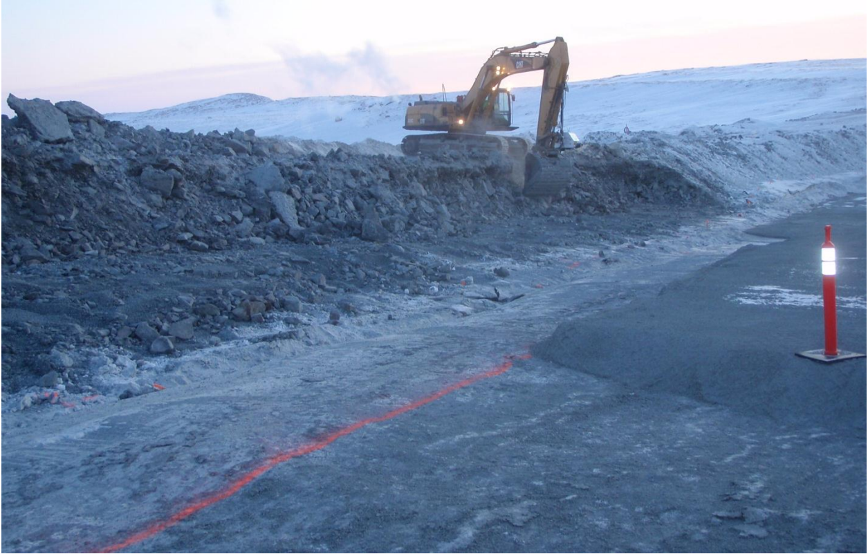
Photo 3: Cat 330 excavator pulling back ROQ on the upstream side of the dam shell.
