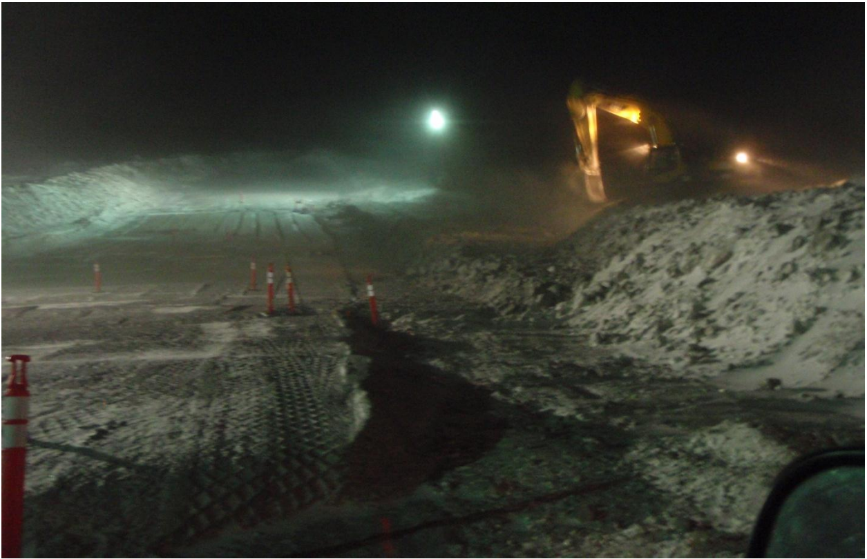
Photo 5: Excavator spreading and shaping ROQ on the downstream side of the dam.
